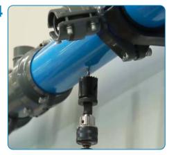
Hold the drill perpendicular to the pipe with the drill bit in the center of the mark placed on the pipe. 05
