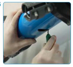
Remove debris and deburr cut edges.
