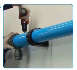
• Tighten the saddle to complete the assembly.
